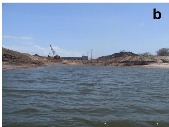
Figure S3. Engineering works (roads, bridges, electrification and housing) associated with the development of wind power fields. Dead mangroves bordering road and bridge crossing a tidal creek are visible (a). Water intake canal construction for aquaculture farms at the main Jaguaribe river. Note remaining mangrove trees to the right behind the dredged material deposition site (b).
